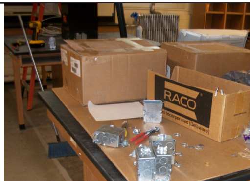
Above, the microbiology lab renovation shows new lab bench. Left, Room 111 showing new benches and shelves. Labs were renovated over the summer, and students began using the improved labs this fall semester.
